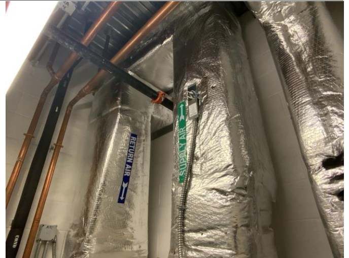
32 - HVAC SYSTEM DUCTWORK
