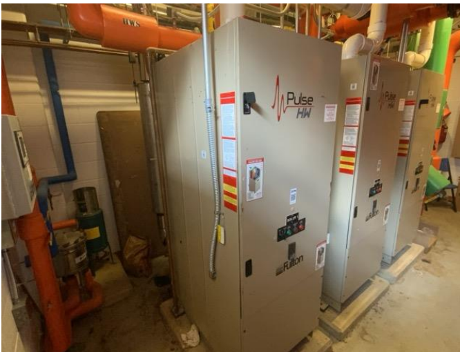
21 - GAS BOILERS IN NEW BOILER ROOM
