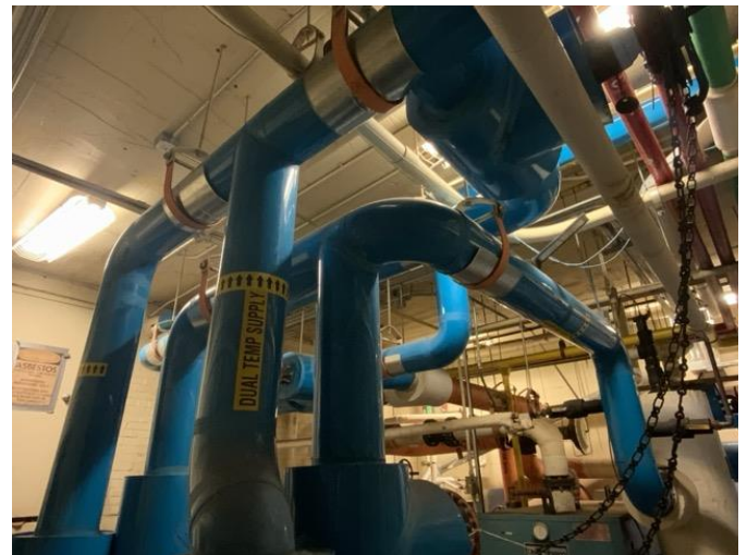
28 - HVAC SYSTEM HYDRONIC PIPING
