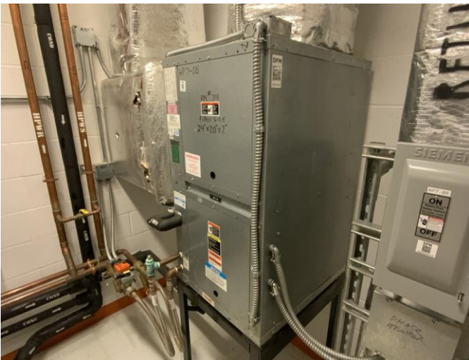
27 - WATER SOURCE HEAT PUMP
